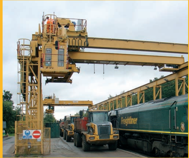
Calvert Landfill in Buckinghamshire. United Kingdom
