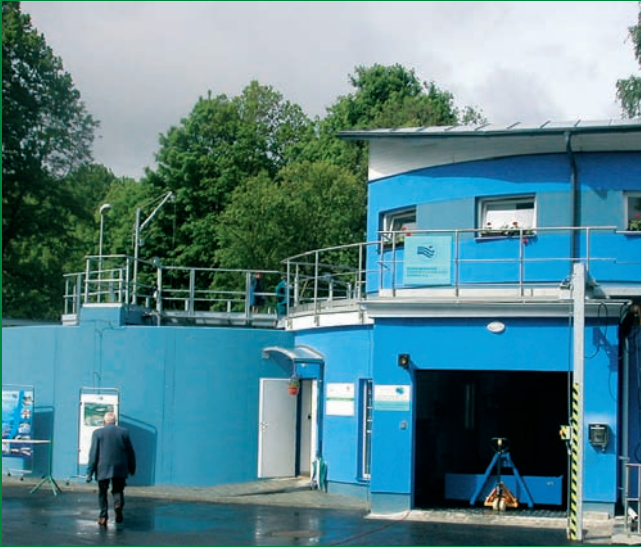
SmVak. Water management. Czech Republic
