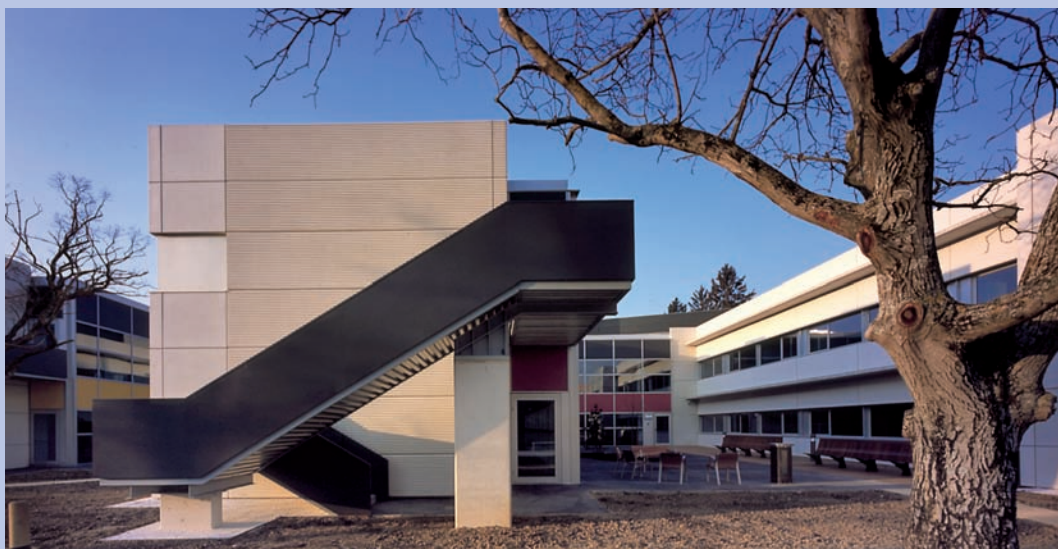
Centre for the mentally handicapped, Pamplona, Navarra
