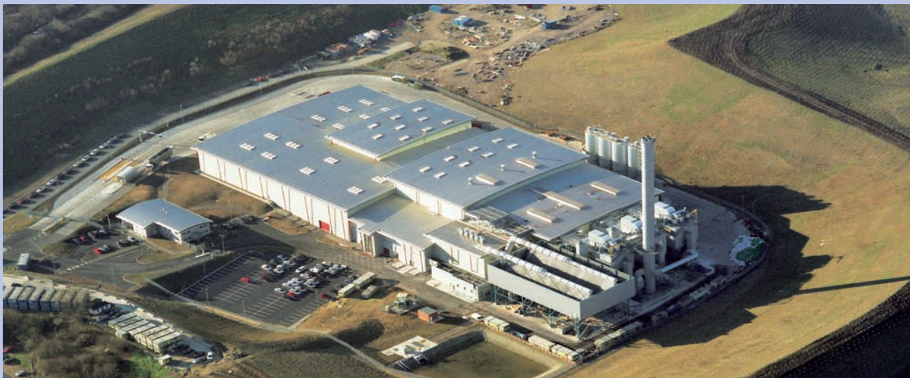
Thermal waste treatment plant. Alington, United Kingdom.
