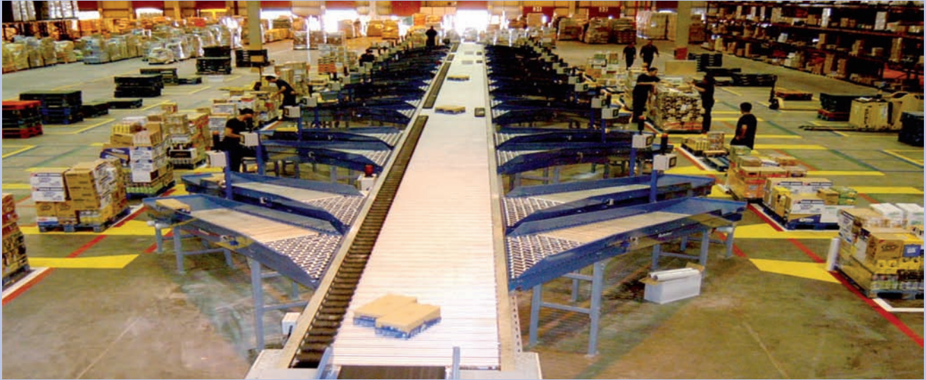
Logistics. Automatic packaging collator in Carrefour warehouse. Seville
