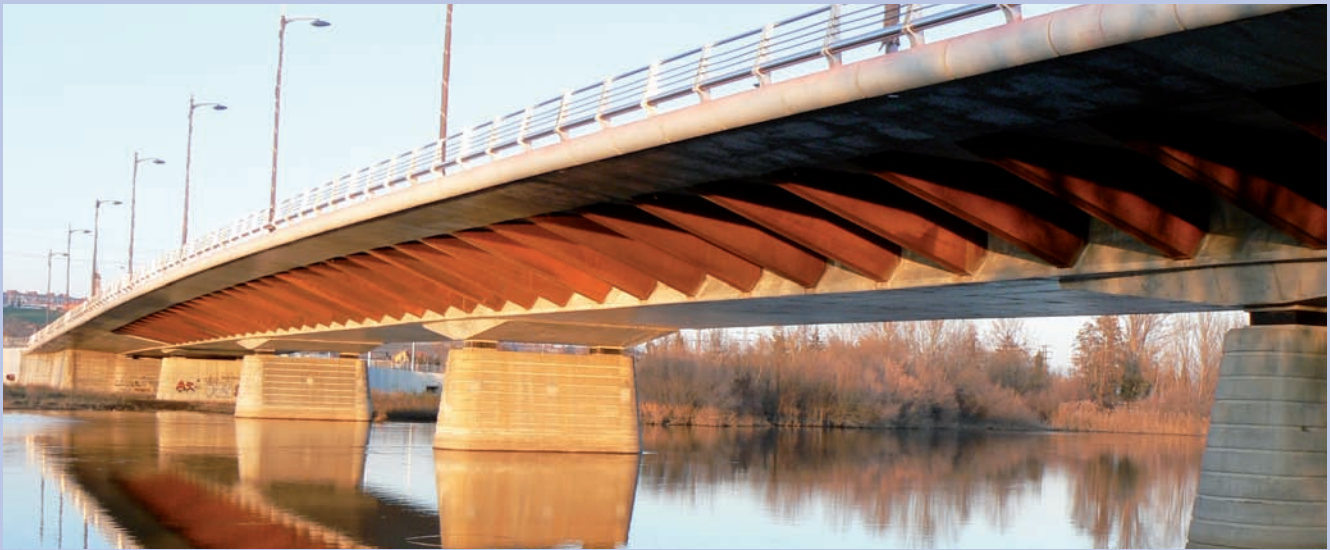
La Serna Bridge, Salamanca
