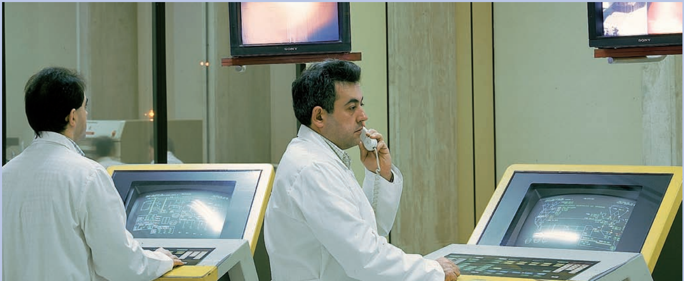
Cement factory control room in Olazagutia, Navarra
