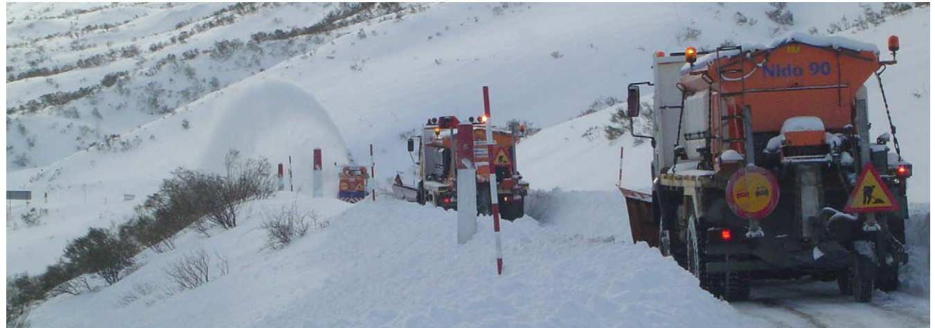
Conservation and maintenance work.
