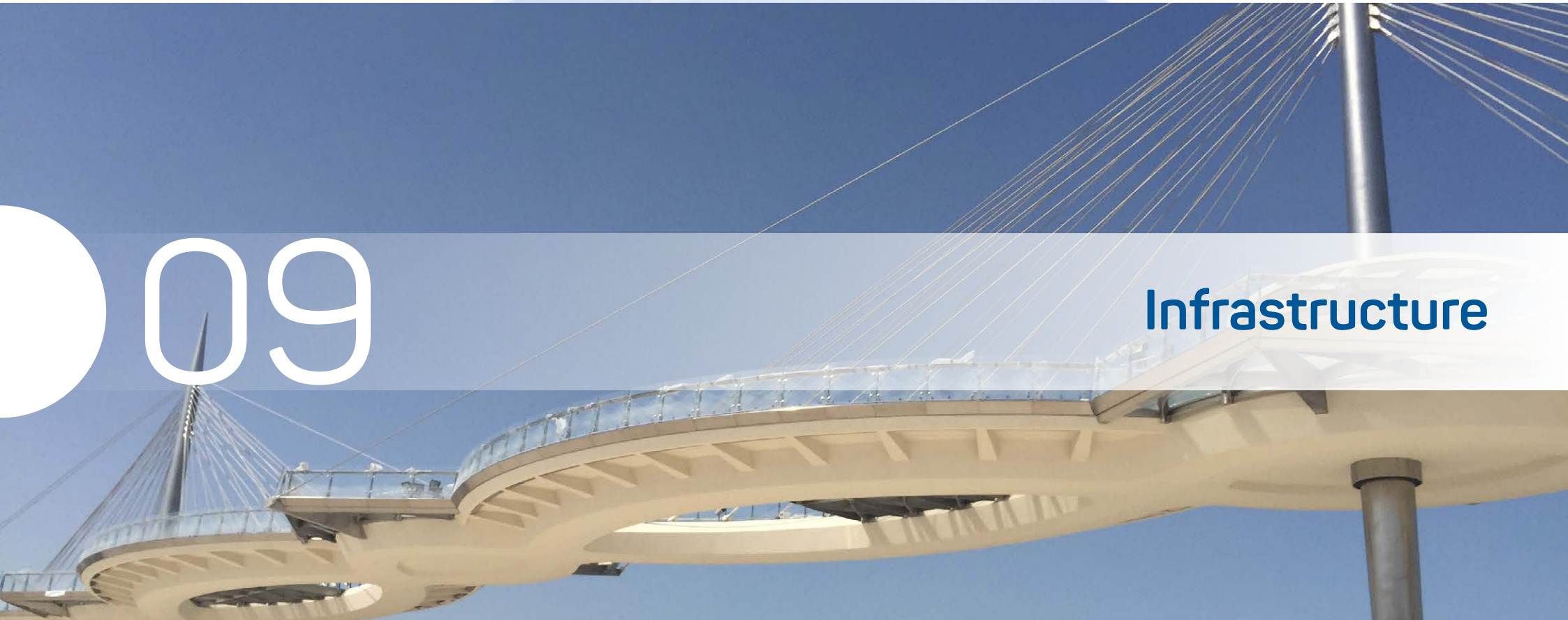
Lusail Pedestrian Bridges (Qatar).
