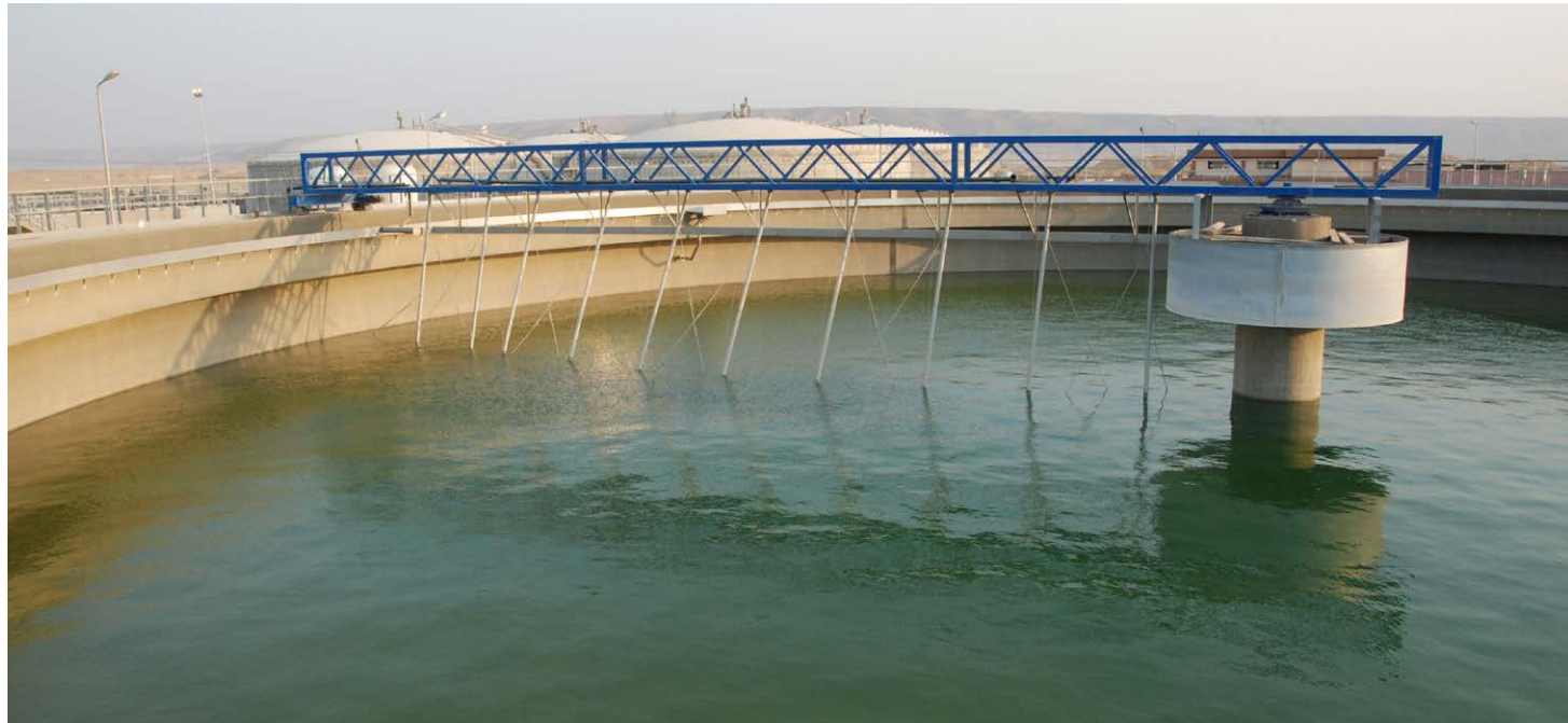
New Cairo Wastewater Treatment Plant (Egypt).
