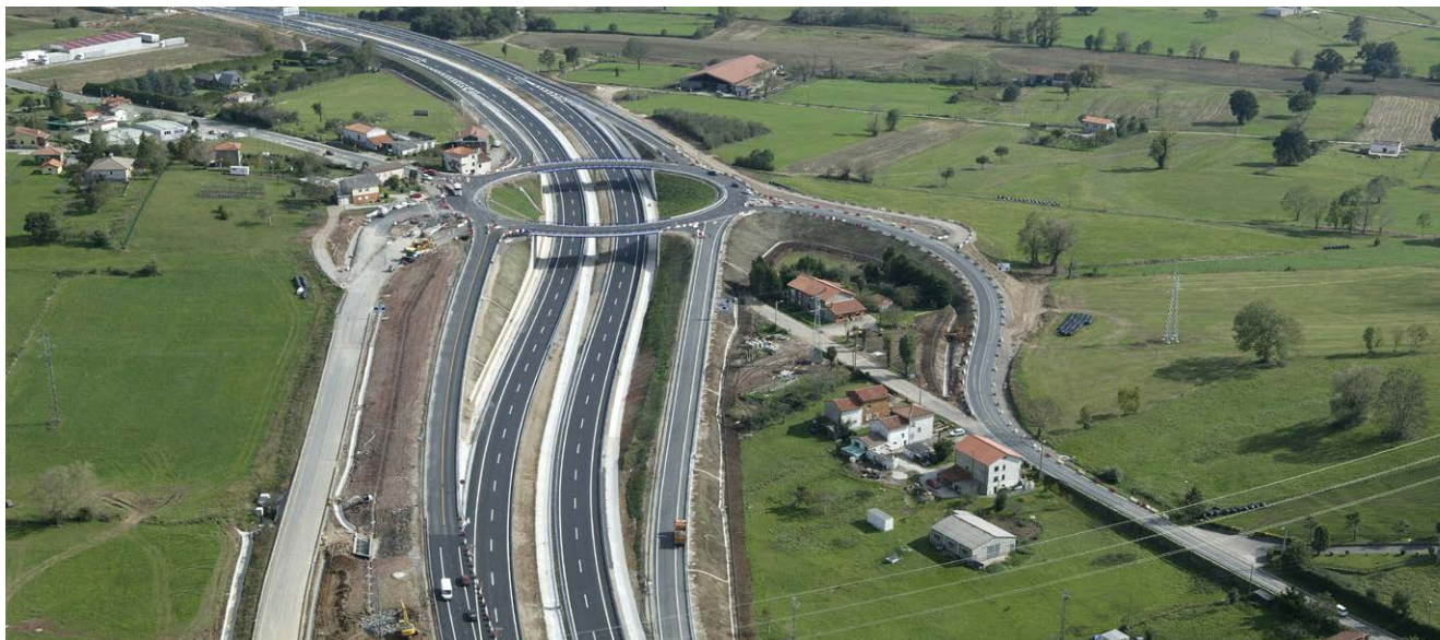
A-8 Dual Carriageway, Solares-La Encina section. Cantabria (Spain).
