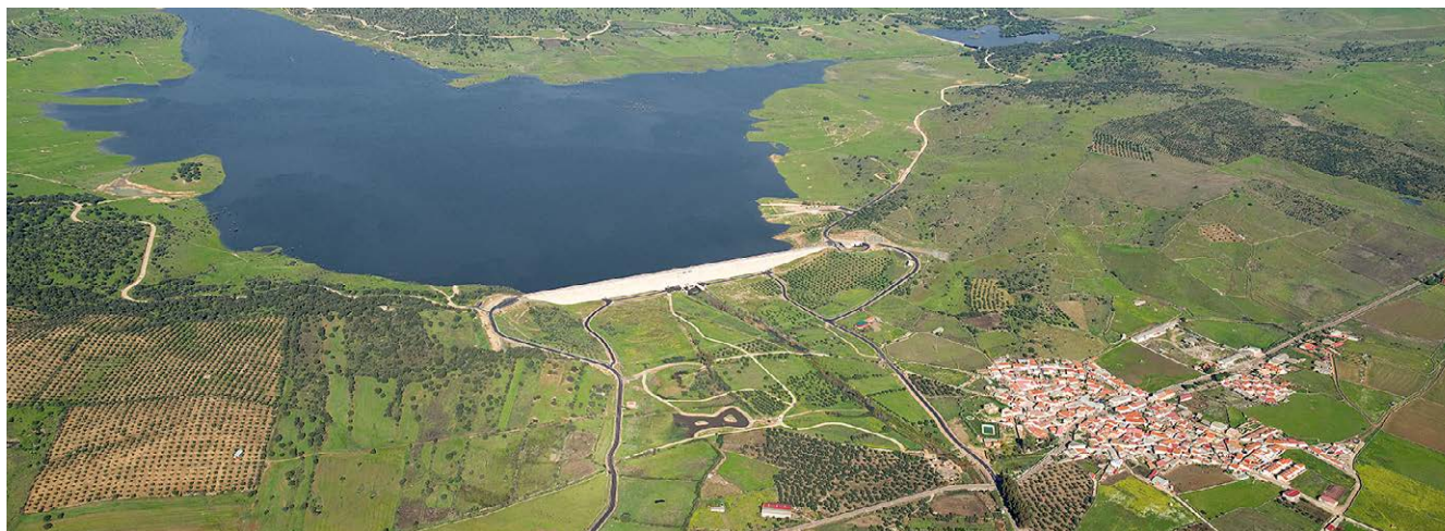
Alcollarín Dam. Cáceres (Spain).
