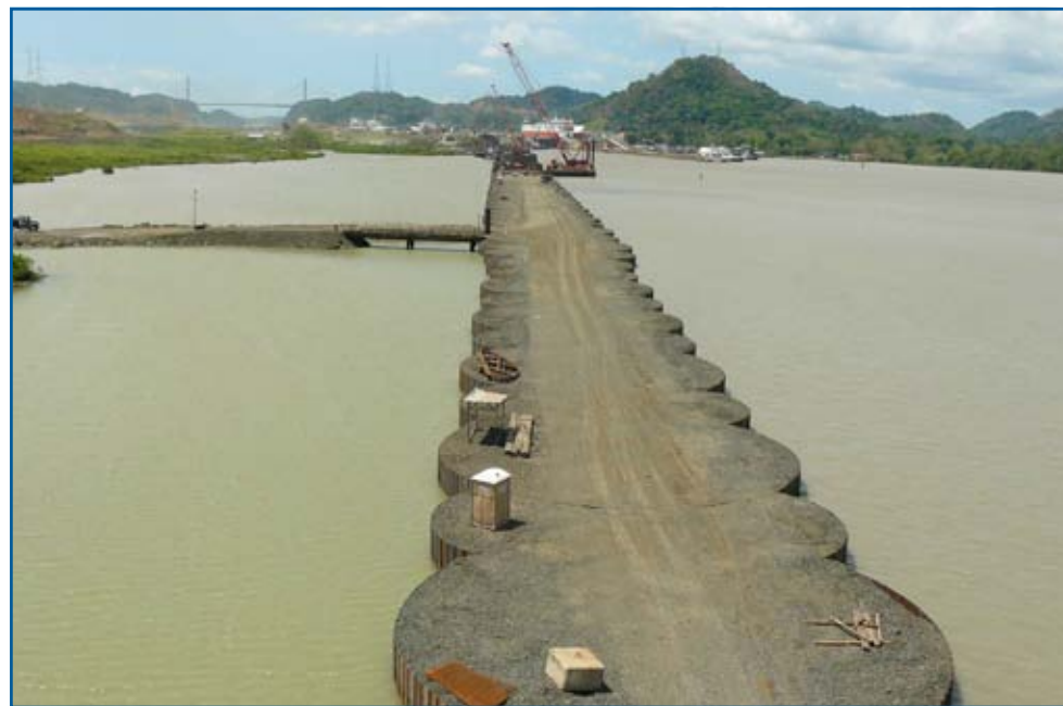
Construction of the Pacific Ocean access channel to the Panama Canal
