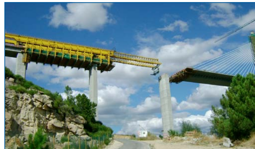
Corgo Viaduct, Portugal
