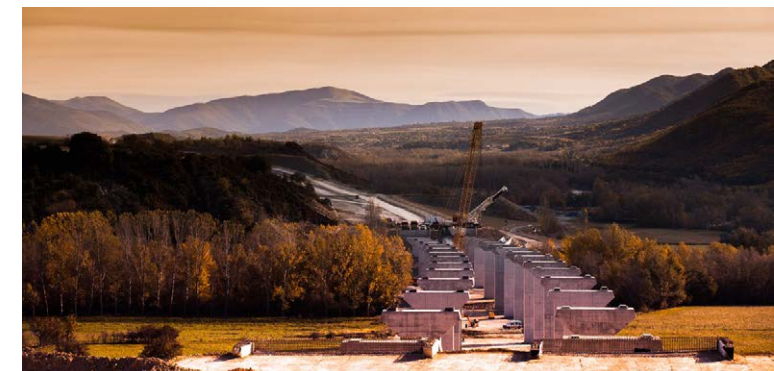
Assembly of beams on the A21 motorway viaduct.
