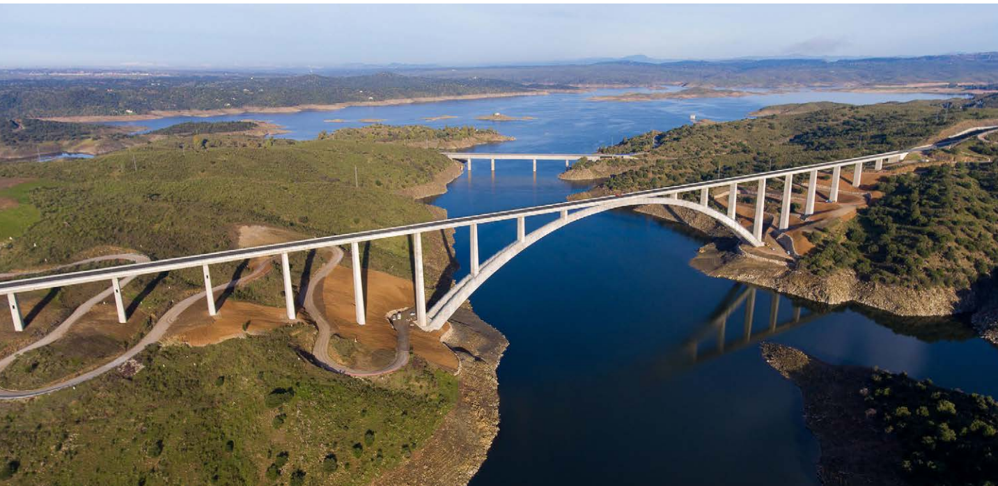
Rio Almonte viaduct, Spain.
