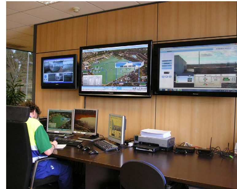
Zaragoza control centre, Spain.
