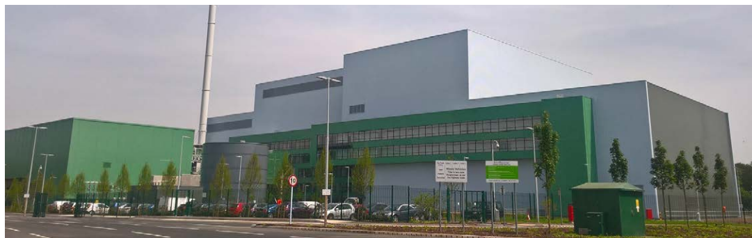
Energy Recovery Centre of Mercia Envirecover, United Kingdom.
