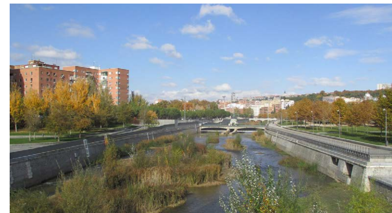
Restoration River Manzanares, Spain.
