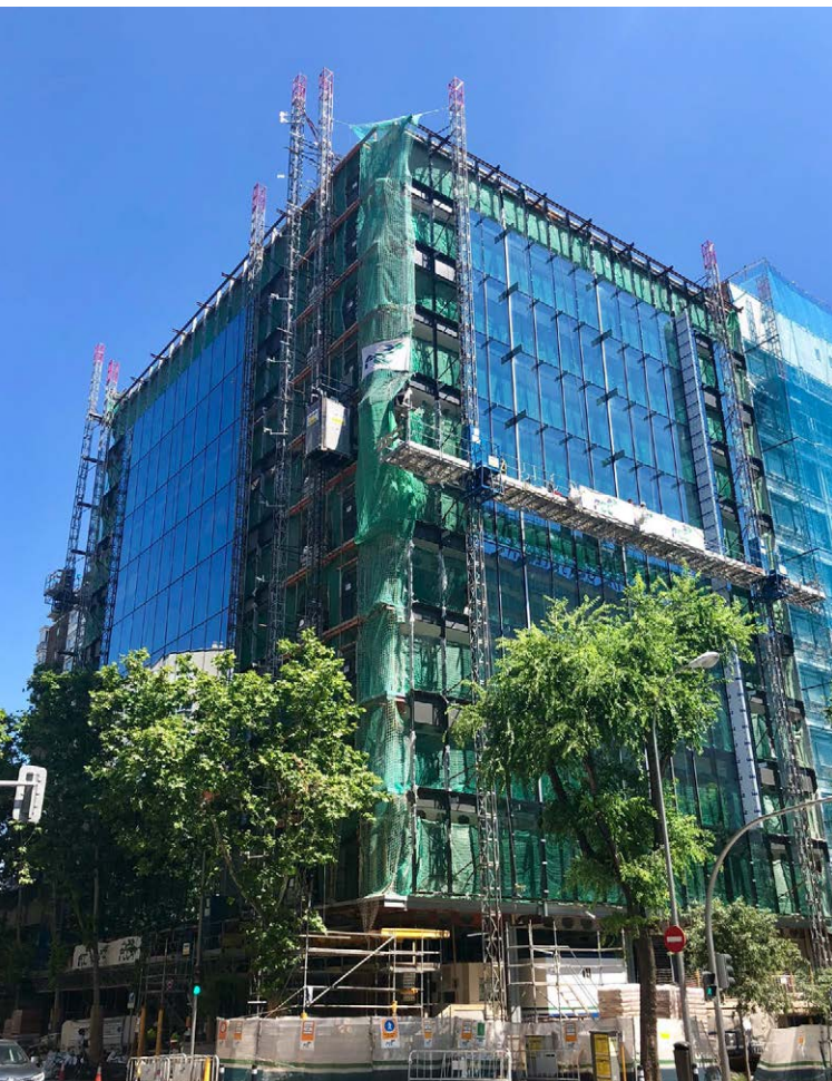
Renovation of the Gorbea 1 building, Madrid.
