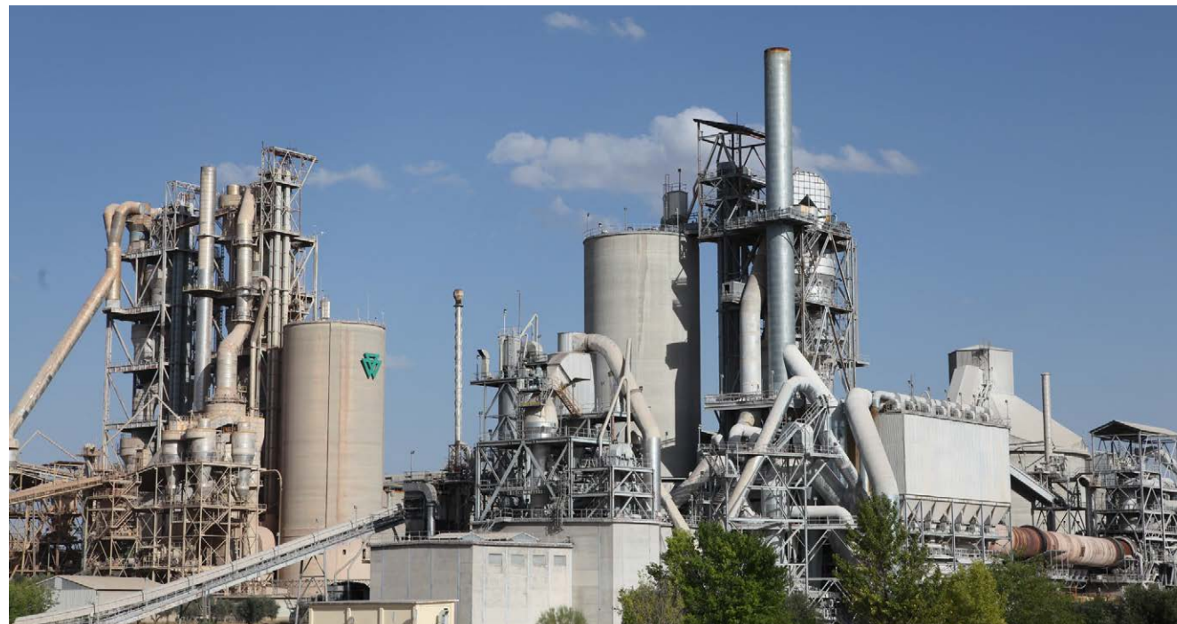
White cement production line. El Alto cement production centre, Madrid.
