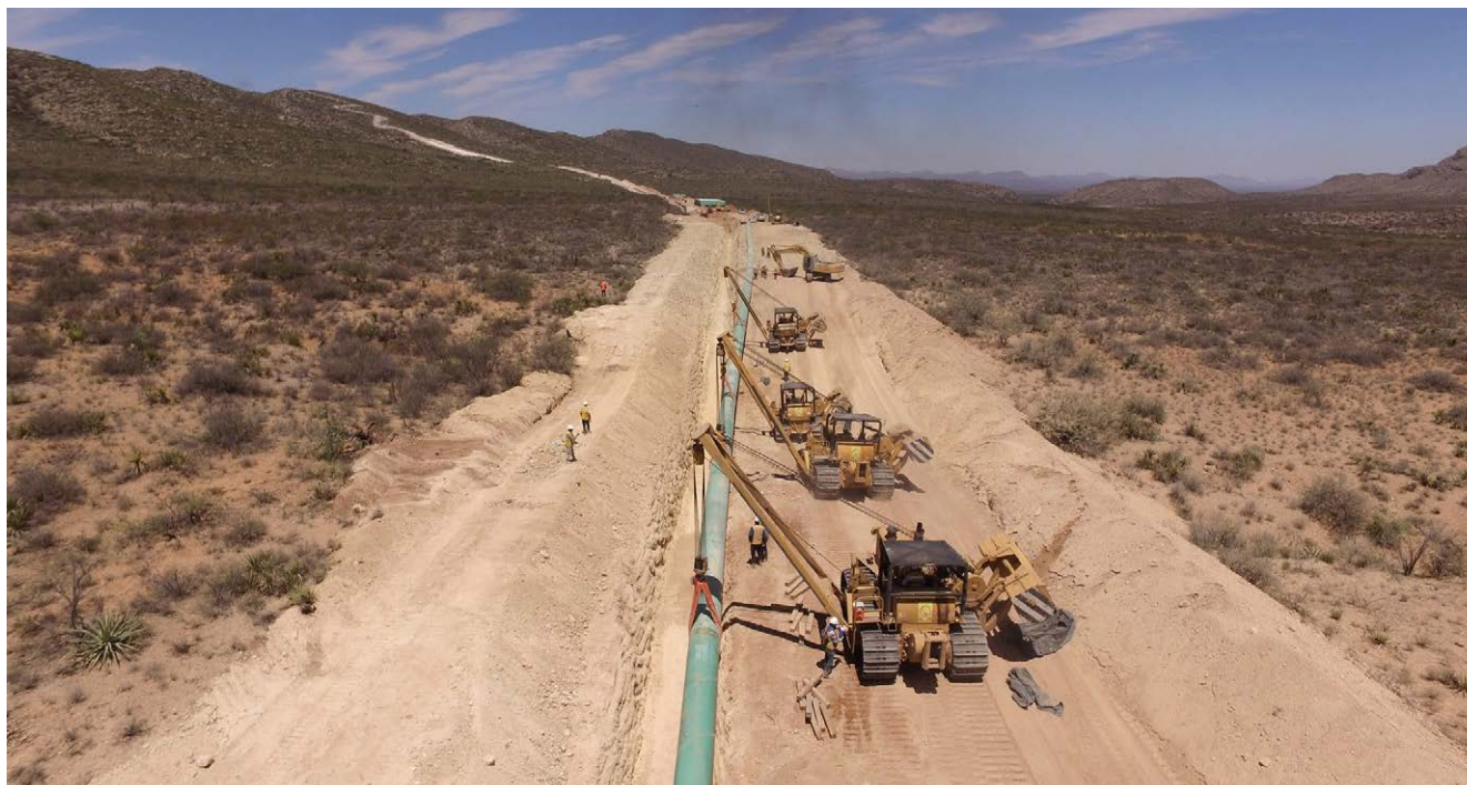
Samalayuca-Sasabe gas pipeline, Mexico.
