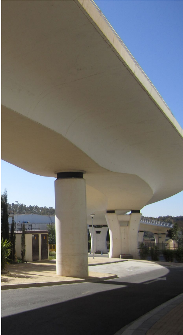
White cement viaduct in Seville (Spain).
