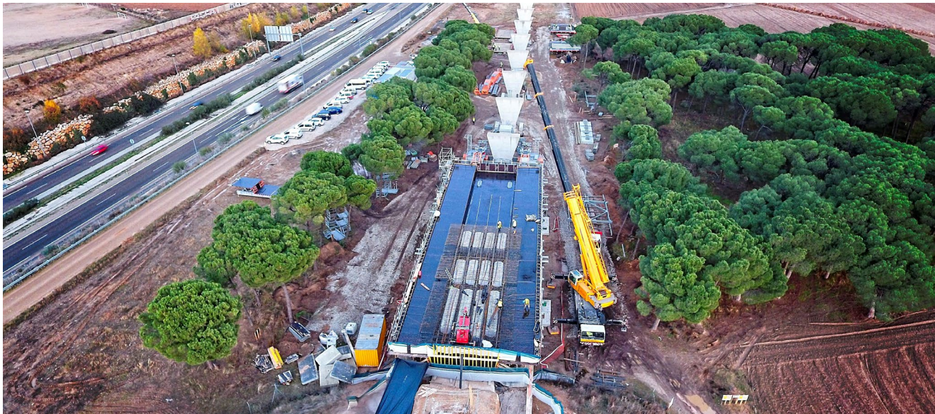
East diversion (Valladolid, Spain).
