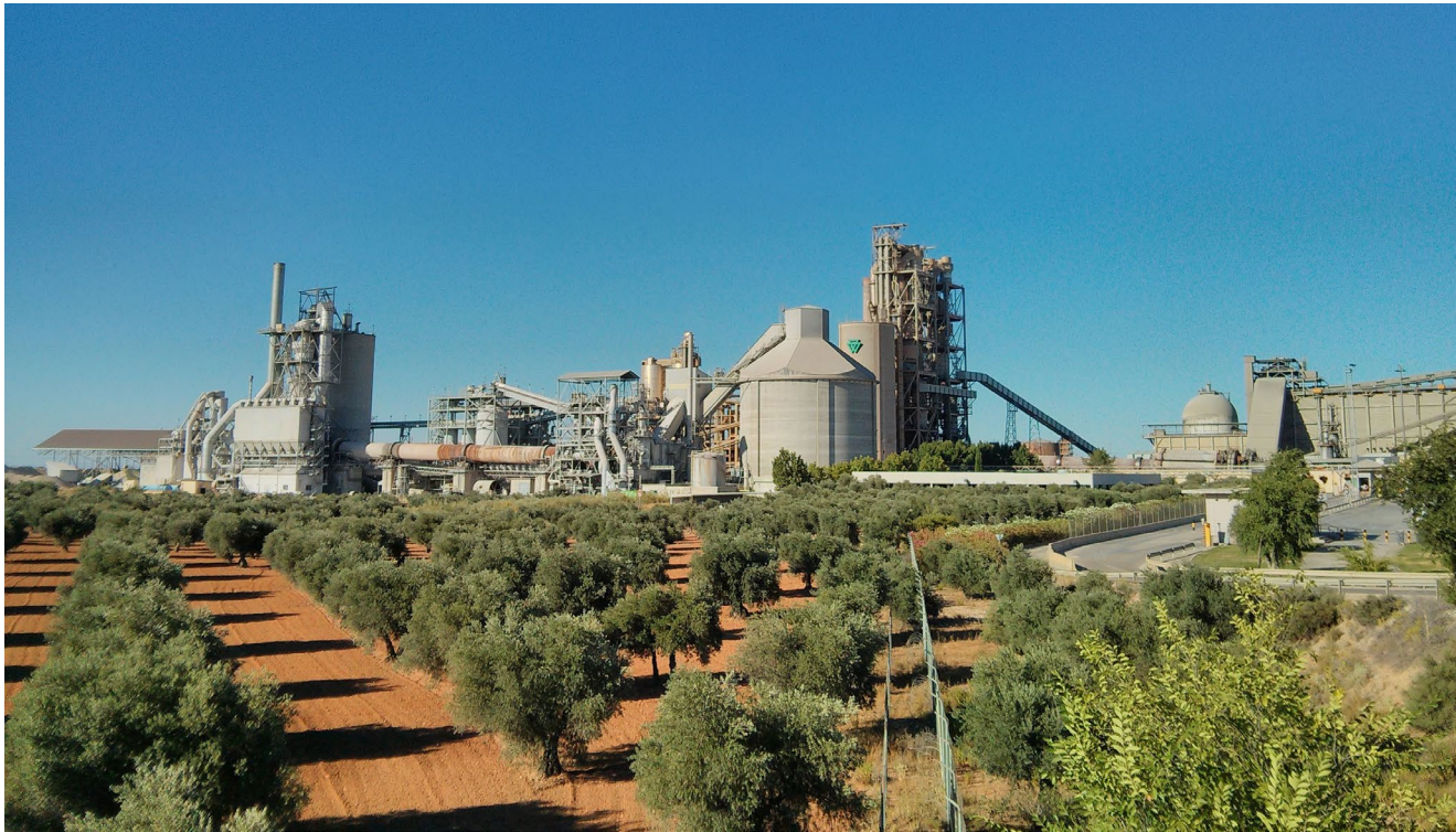
Panoramic view of the factory in El Alto, Morata de Tajuña (Madrid, Spain).
