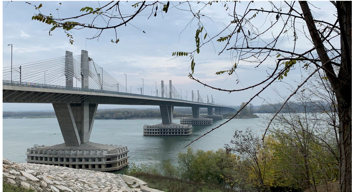
Bridge over the Danube river, between Vidin (Bulgaria) and Calafat (Romania).
