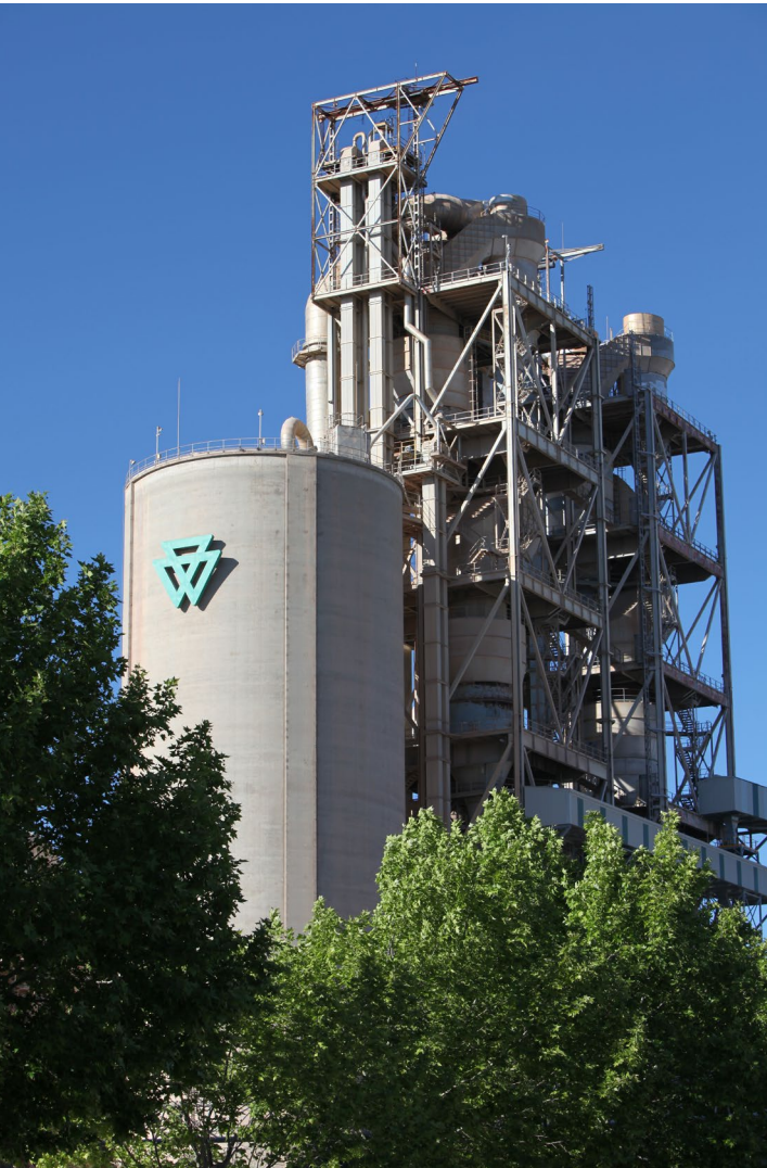
Pre-calcination tower at the factory in El Alto, Morata de Tajuña (Madrid, Spain).
