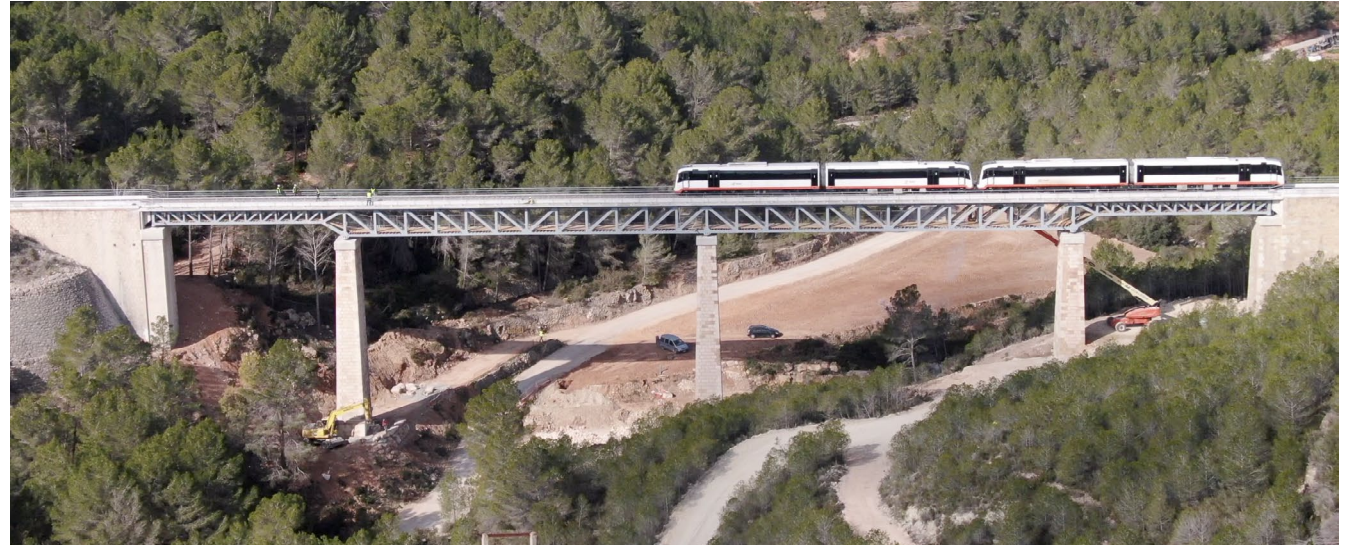
Ferrandet viaduct (Alicante, Spain).
