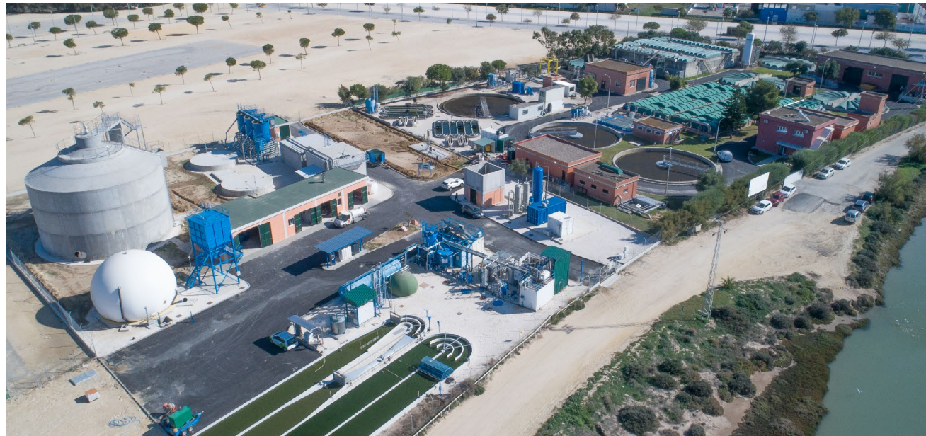
H2020 Incover Project. Chiclana WWTP in Cadiz (Spain).
