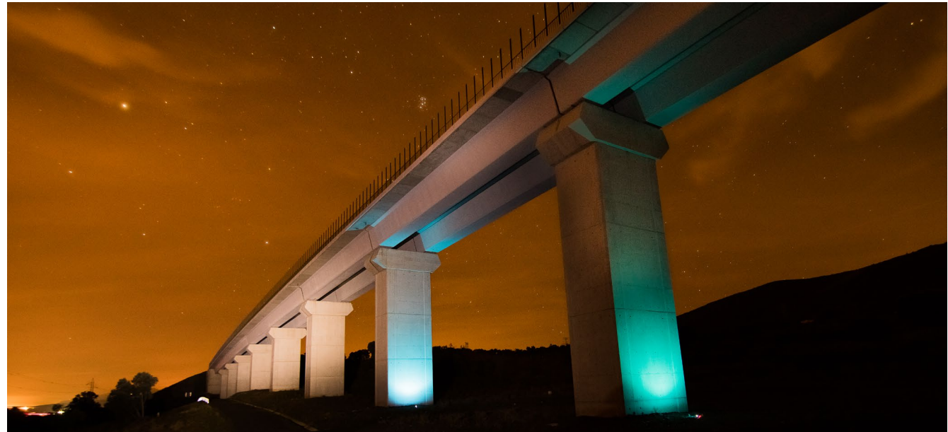
Rivero Viaduct. Trackbed of the High-Speed Madrid-Extremadura Line. Talayuuela-Cáceres. Section: Arroyo de la Charca-Grimaldo (Cáceres, Spain).
