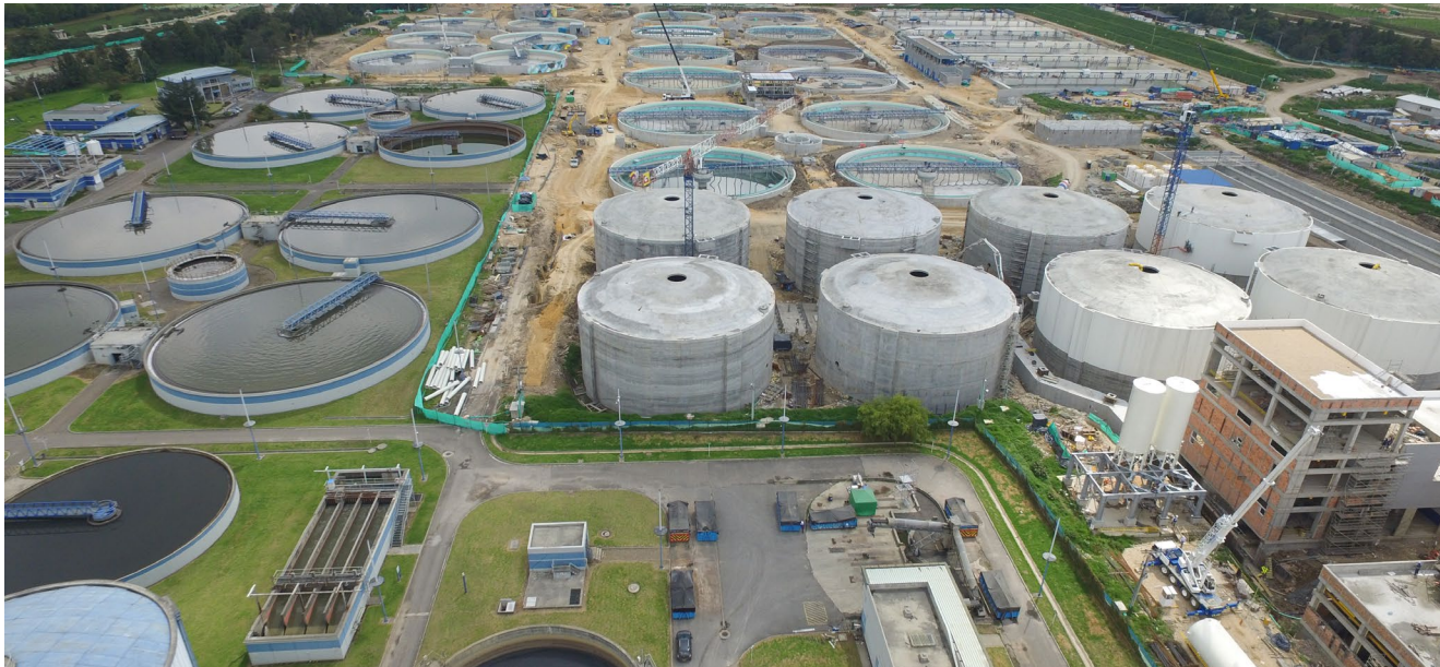
"El Salitre" wastewater treatment plant in Colombia.
