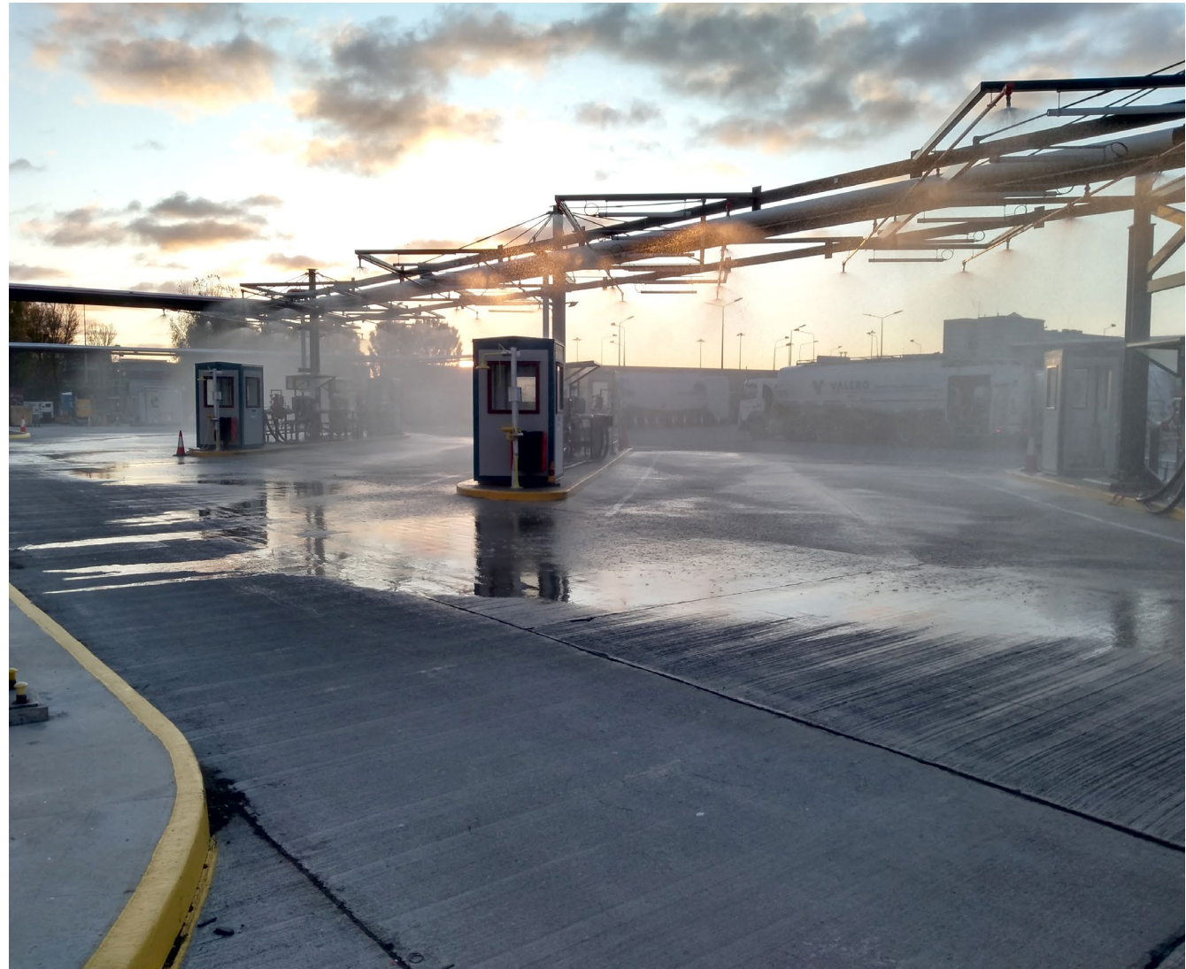
Remodelling of airport and fire hydrant system in Dublin Airport (Ireland).
