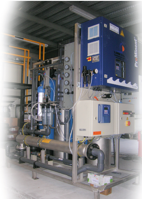
Recycled shower water for use in laundry facilities.
