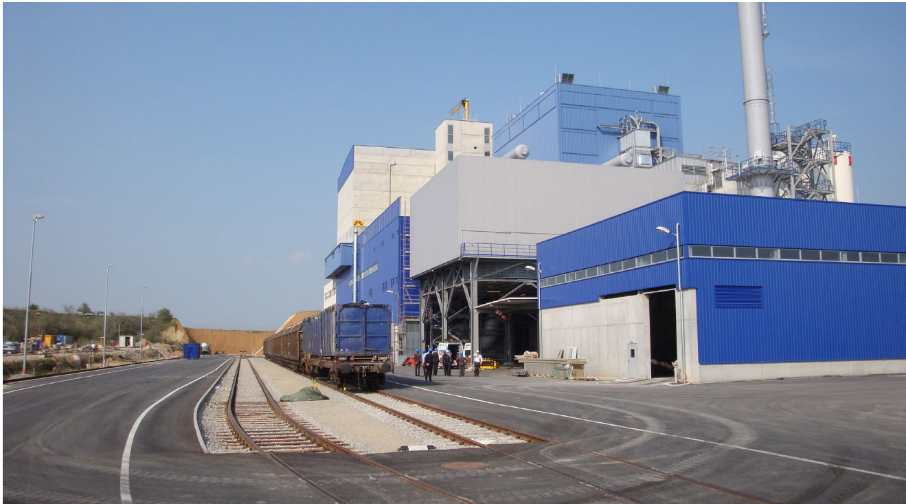
Urban solid waste energy recovery plant, Zistersdorf (Austria).
