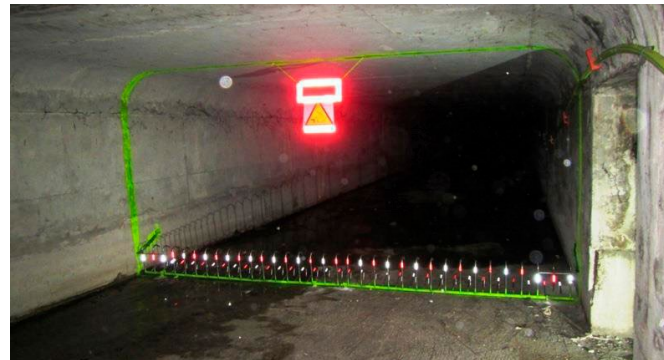
Comb separator in sewer systems Barcelona.
