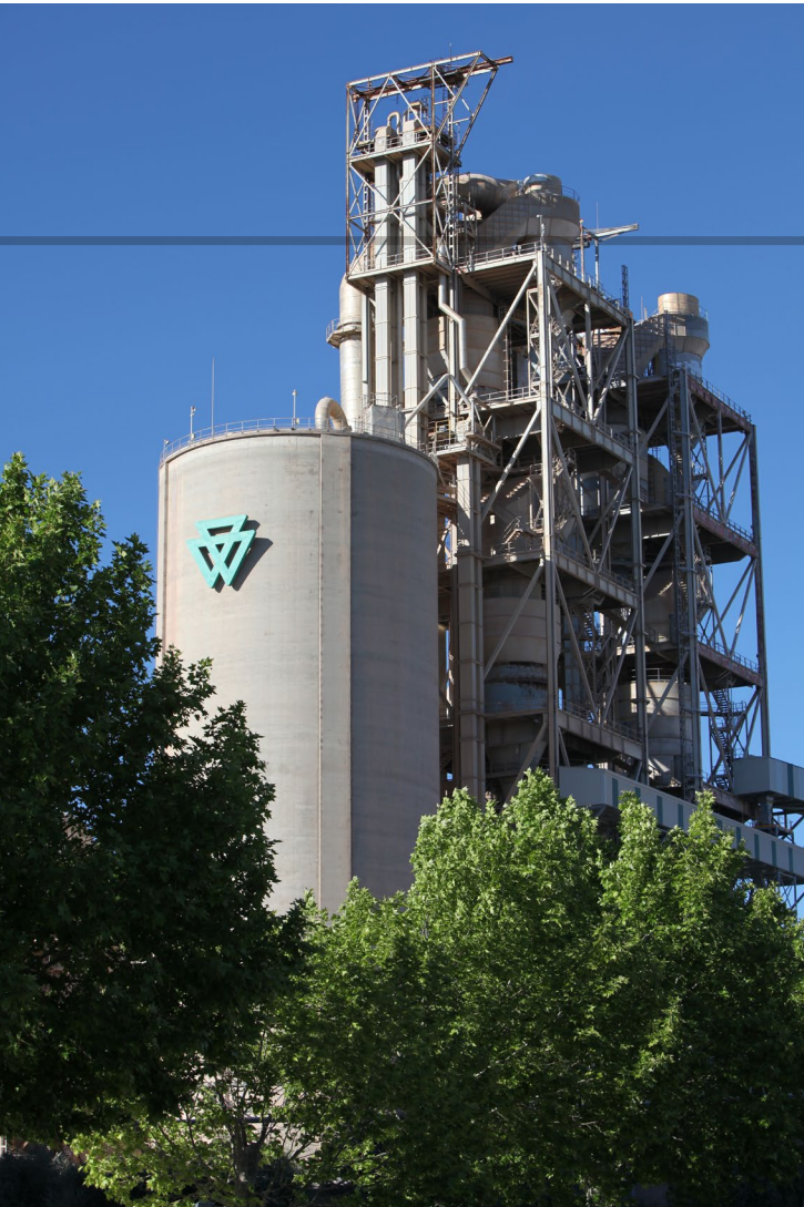
Precalciner tower. El Alto factory, Madrid (Spain).
