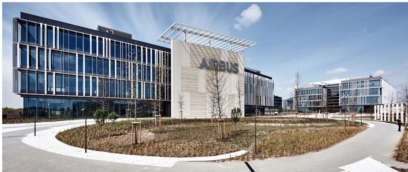
New corporate headquarters "Campus Airbus Futura", in Getafe (Madrid, Spain).
