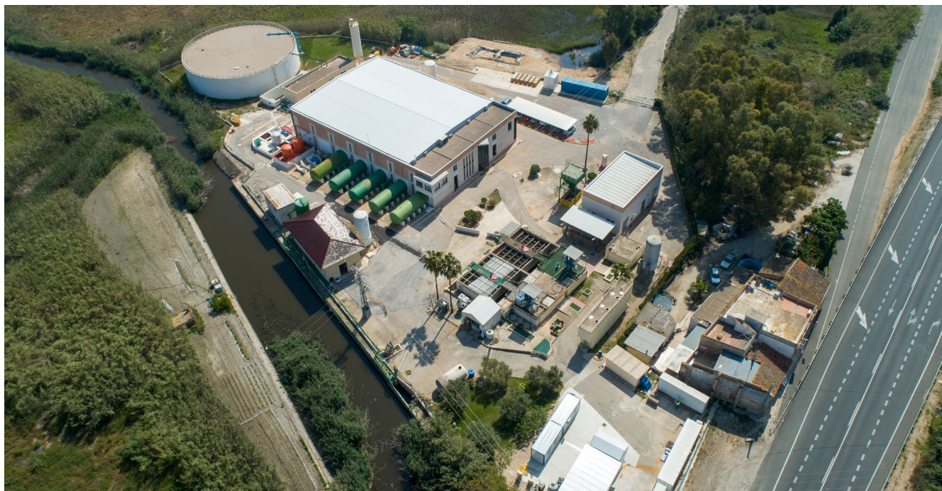
The MIDES project, led by Aqualia, operates the first two desalination plants that are wholly energy self-sufficient in the world, in Dénia (Alicante, Spain) and Guía de Isora (Santa Cruz de Tenerife, Spain).
