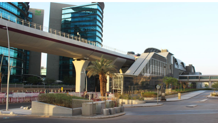
Lines 4-5-6 of Riyadh Metro (Saudi Arabia).
