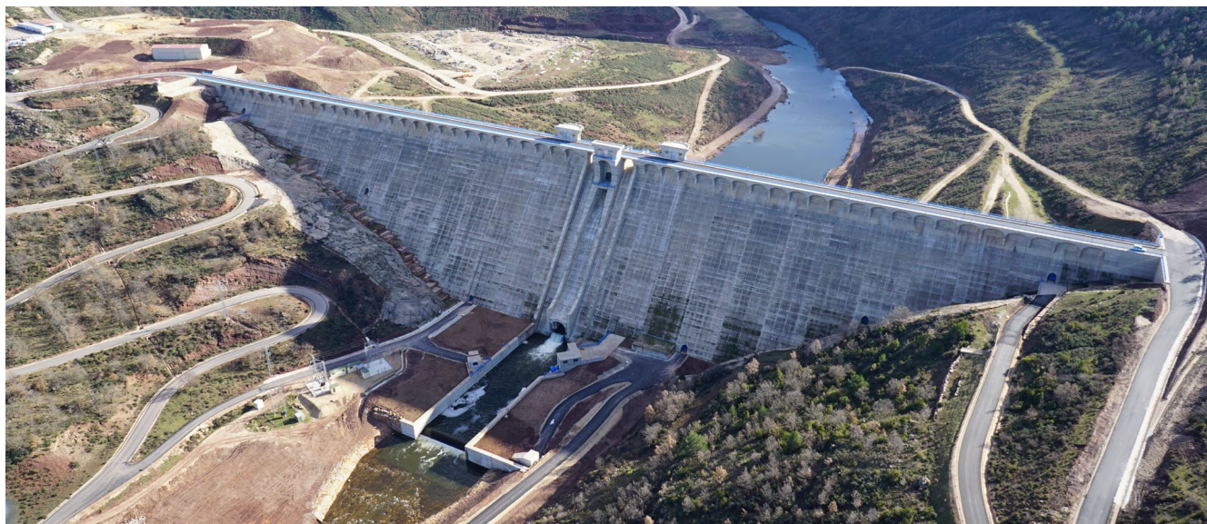
Castrovido Dam, Burgos (Spain).
