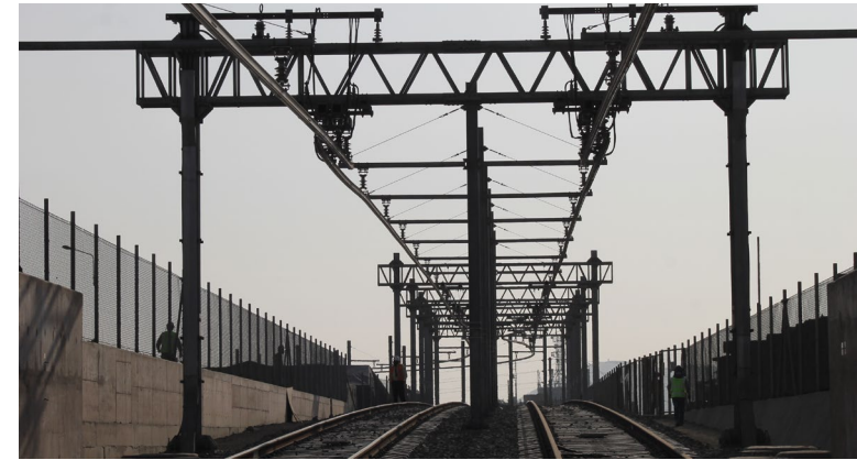
Line 2 and branch line 4 of Lima Metro (Peru).
