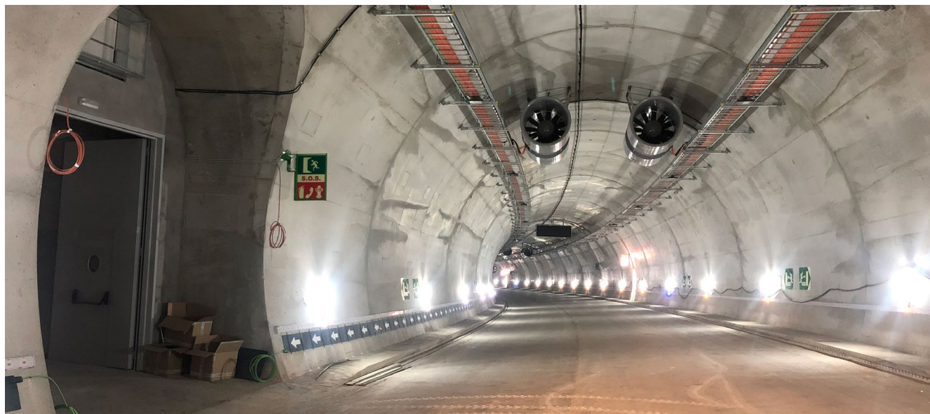
Vallirana tunnel, Catalonia (Spain).
