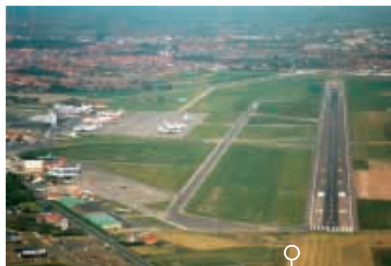
AERIAL VIEW of the Ostend-Bruges airport facilities.
