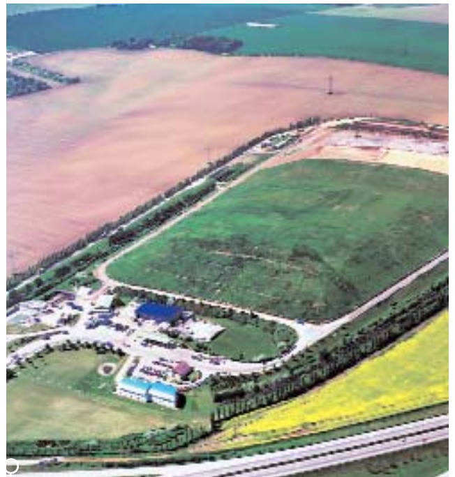
IN THIS PAGE, THE WASTE DUMPING SITE AT ZABCISE, Czech Republic. On the page on the right, a street sweeper vehicle in Brno, the Czech Republic's second largest city, and a biological waste treatment plant in Halvenrain, Austria.
