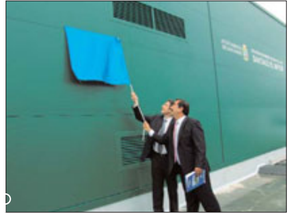
INAUGURATION OF the general drainpipe in the San Martín District by the mayor of Santander, Gonzalo Piñeiro and the secretary for the Environment, Íñigo de la Serna.
