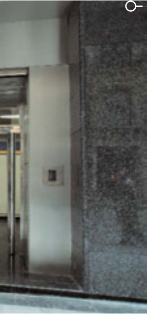
NEW ACCESS AND vestibule at the Sol metro station, with access from a commercial centre.
