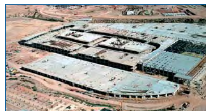
Aerial view of the Commercial Centre.
