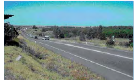
The current section of the road where the project is to commence. Above, Juan Carlos Rodríguez Ibarra, President of the Extremadura Autonomous Community, lays the first stone for the new access road to Badajoz from the Cáceres road.
