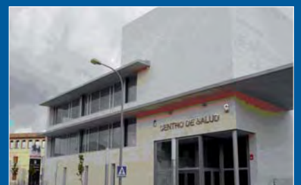
Main entrance of the Healthcare centre. Above, the President of Castilla-La Mancha during his visit to inaugurate the facilities in Casas Ibáñez, Albacete.
