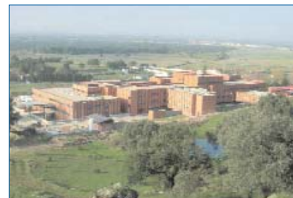
The refurbishment doubled the hospital's useful floor space.
