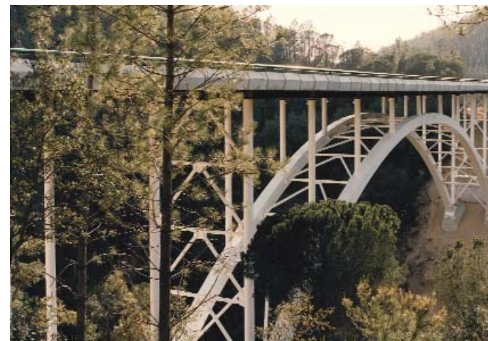
On the left, the current Transversal Catalu a-Lleida-Girona road: Camins-Santa Coloma-Girona section, built by FCC in 1995. Above, Les Fosses Bridge, winner of the Construmat award for the best civil works in 1997.
