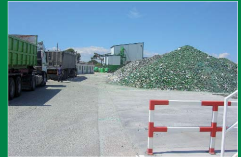
On the top, the glass treatment plant in Cadrete in Zaragoza. On the left, the facilities in Muel in the same province.
