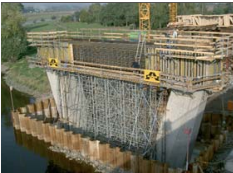
Below, work on the 366 metre-long bridge.
