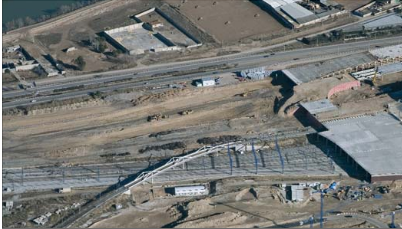
Aerial view of the work site near Delicias Station in Zaragoza
