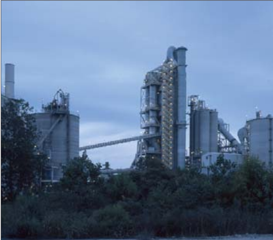
The cement plant in Harleyville, South Carolina, United States of America.
