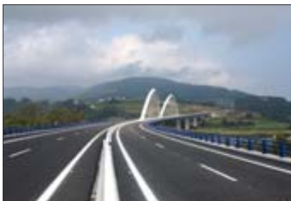
Above, Canero viaduct in the Cantabrico Highway at the Querúas-Otur stretch. Above these lines, detail of the Navia relief road.
