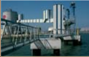
Cementos Alfa inaugurates new Raos Harbor facilities in Santander. Page 34
