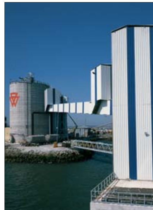
The silo, with a diameter measuring 19.60 meters and a height of 29.60 meters, is a structure built with reinforced concrete
