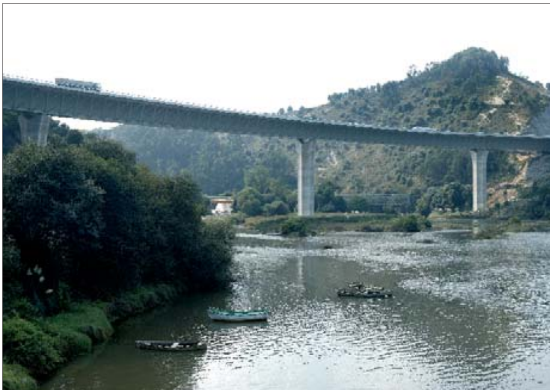
Above, the Acebo viaduct in the Caravia-Llovio stretch of the highway. Above these lines, the viaduct across the Tina Menor inlet, part of the Lamadrid-Unquera highway section.
