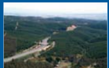
The first two images are of the SCADA toll motorway (Autopista de Aconcagua), part of Route 5, better known as the Pan-American Route, the country's most important major road stretching from the north to the south of Chile. Above these lines, another image of the Itata Toll Motorway.
