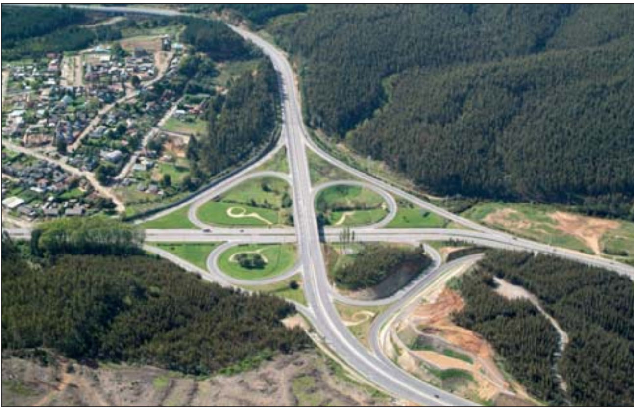
The 89 Km long Autopista SCADI, Autopista de Itata, is in the southern part of the country, at an approximate distance of 600 Km from Santiago de Chile from the northern access at Concepción, one of the country's regions showing the strongest industrial and forestry growth.
