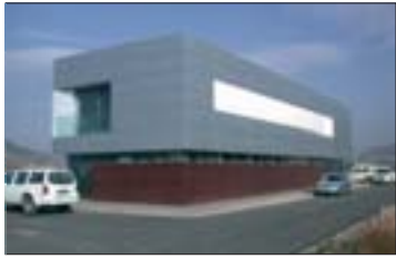
The Puig Reig-Berg (Barcelona) tunnel control building.
