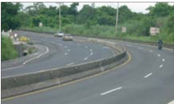
The Pan American Road connects the cities of Arraiján-La Chorrera in the western region of Panama.
