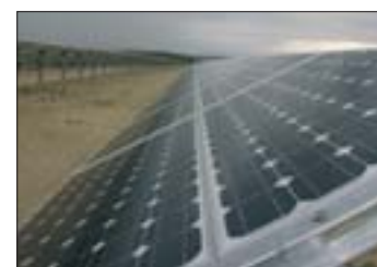
Above, the Cortijo Viejo photovoltaic park. Above these lines, the Sierrasita park
